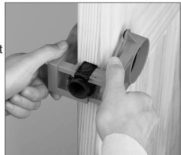
2. Drill Face and Latch Bore Holes
